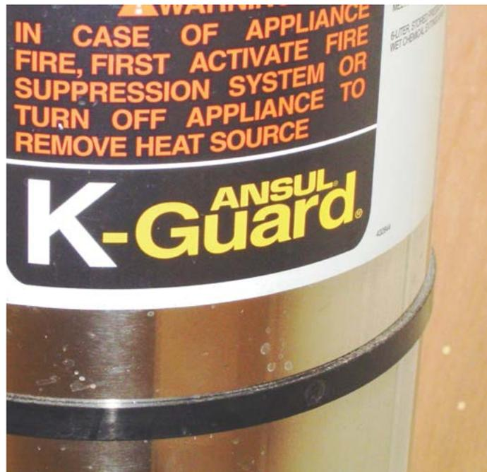
*These pictures are of a portable K-rated fire extinguisher. A class K fire extinguisher is designed to better control grease and other kitchen-related fires. If a kitchen contains any grease-producing appliances, a portable Class K-rated fire extinguisher should be installed in the kitchen in a visible and easily accessible location.*
