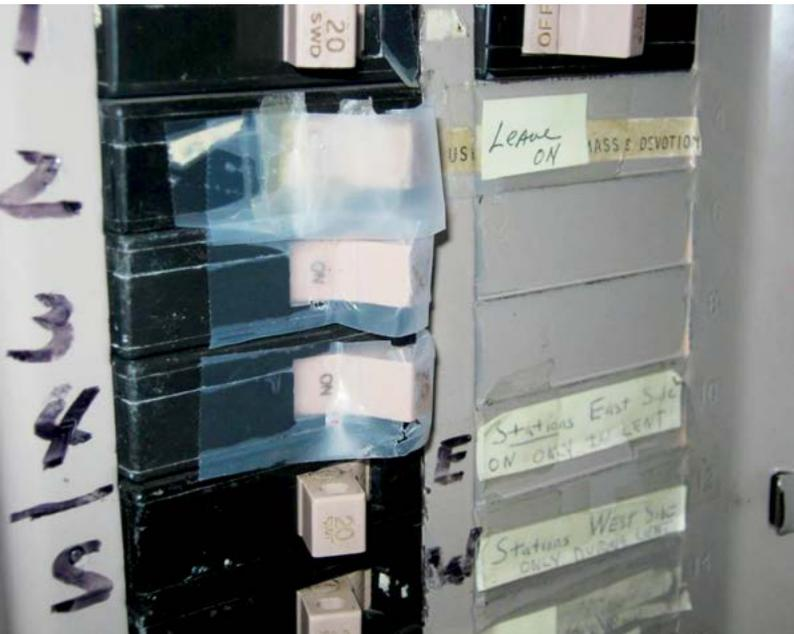
The image above shows breakers taped in the ON position. This practice should never be done.
