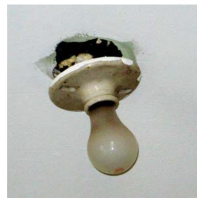
Bottom left: This image shows a broken light fixture. This exposes the wiring to physical damage, dust, dirt and moisture accumulation.
