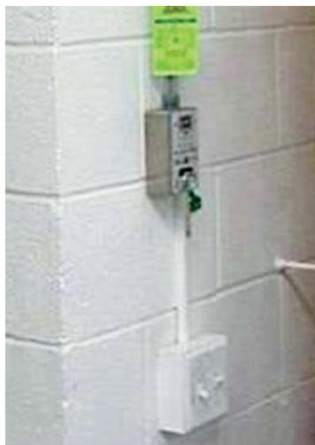
These photos are examples of manual activators that should be used if the automatic extinguishing system fails to activate. Such devices should be installed away from the cooking surface, next to an entrance/exit for the kitchen. Kitchen staff should be aware of this manual activator and trained on its use. Also note the inspection tag. Many fire service companies place these tags on the manual activator to indicate current servicing.
