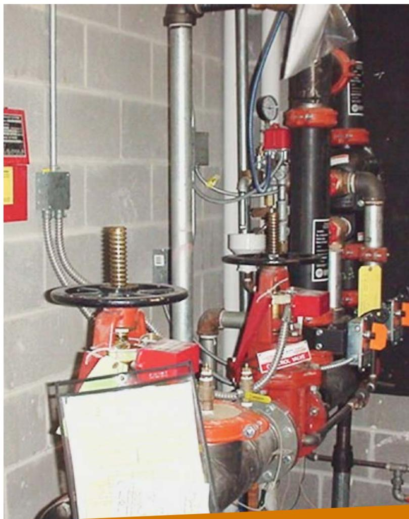
*This photo shows an example of a sprinkler system main valve. Note the inspection report attached to the sprinkler main. The report contains information on the sprinkler system, when it was last inspected and details regarding the inspection.*
