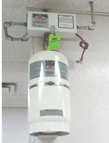
These photos are examples of two different brands of automatic extinguishing systems that contain a liquid extinguishing agent. Ansul and Range Guard are two well known manufacturers. Also, note the inspection tag on the unit to the left. This is the inspection tag that the servicing company will leave after they service the system every six months.
