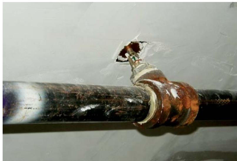
*This photo is an example of a sprinkler head that was installed too close to the wall and would not have an adequate spray pattern.*
